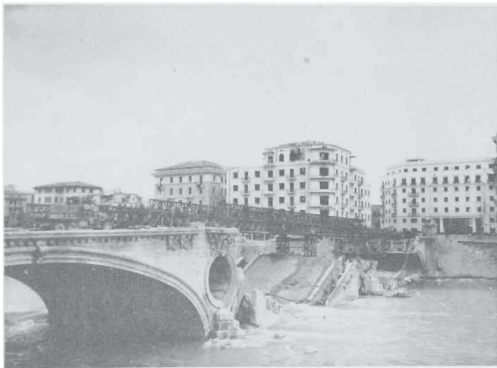
BRIDGE OVER ADIGE BUILT BY 235TH ENGINEERS OF THE 1108TH GROUP
