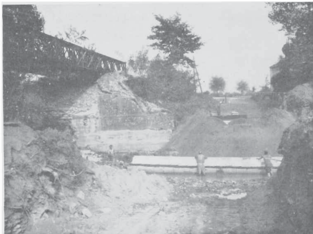
39TH PLACING CULVERT NEAR CAVALLINA
