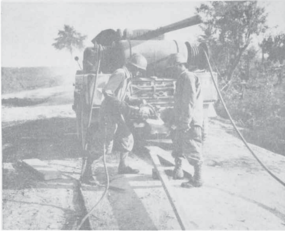
ENGINEERS CUTTING BRIDGE TIMBERS
