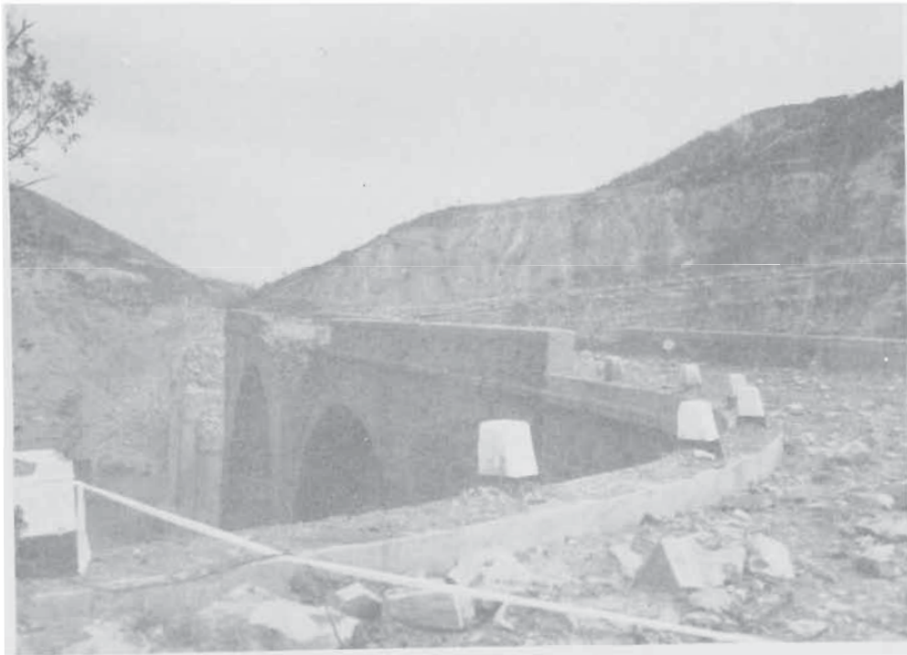
BRIDGE NEAR FIRENZUOLA BYPASSED BY 313TH
