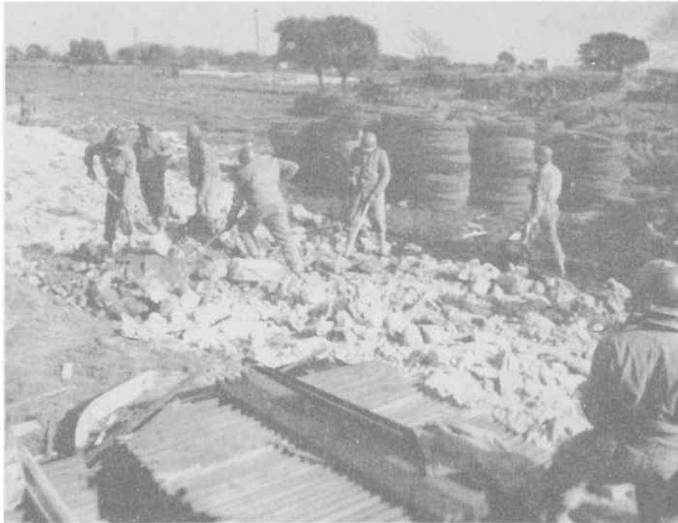
ROAD IN BEACHHEAD ENGINEER DUMP BEING BUILT BY 387TH BATTALION
