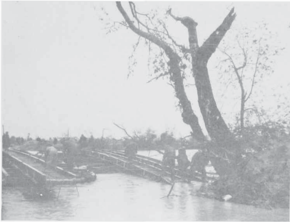
16TH ENGINEERS TRY TO SAVE TREADWAY
