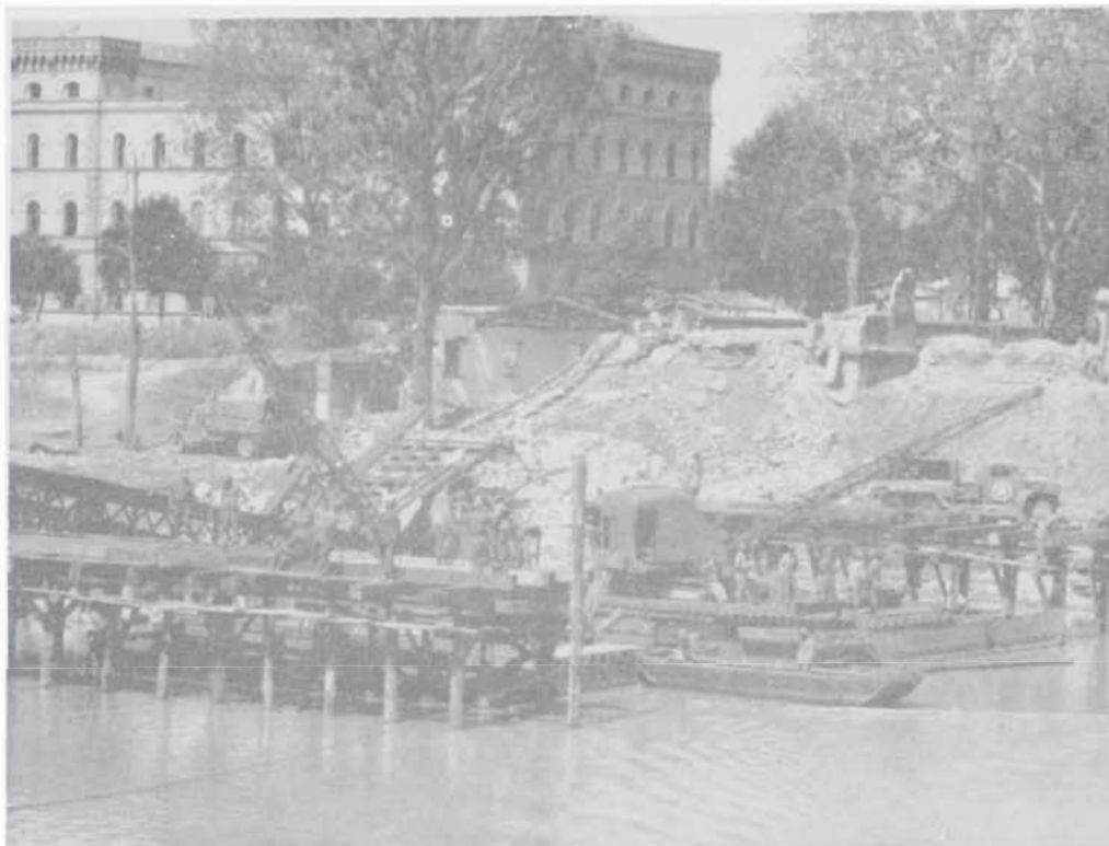
1554TH PONTON RAFT BEING USED IN CONSTRUCTION OF BRIDGE AT FLORENCE
