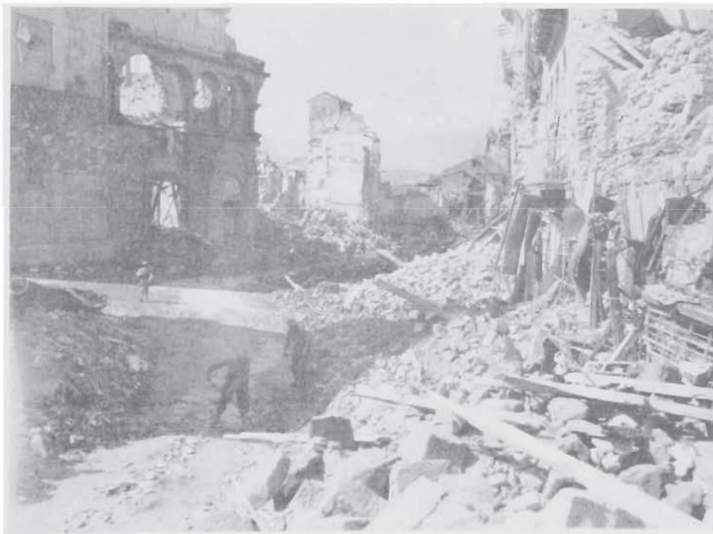
RUBBLE CLEARING OPERATIONS
