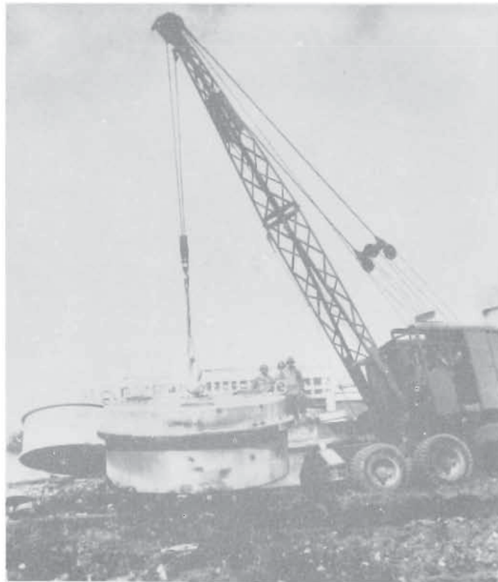
540TH ENGINEERS CLEARING NAPLES
