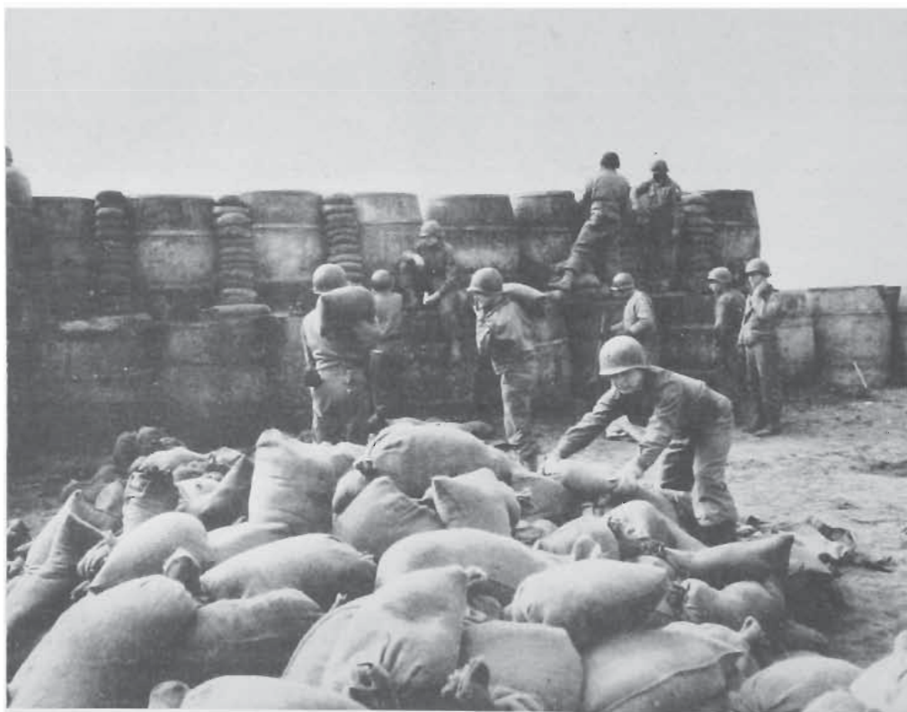
36TH BUILDS AIRPLANE REVETMENTS AT NETTUNO
