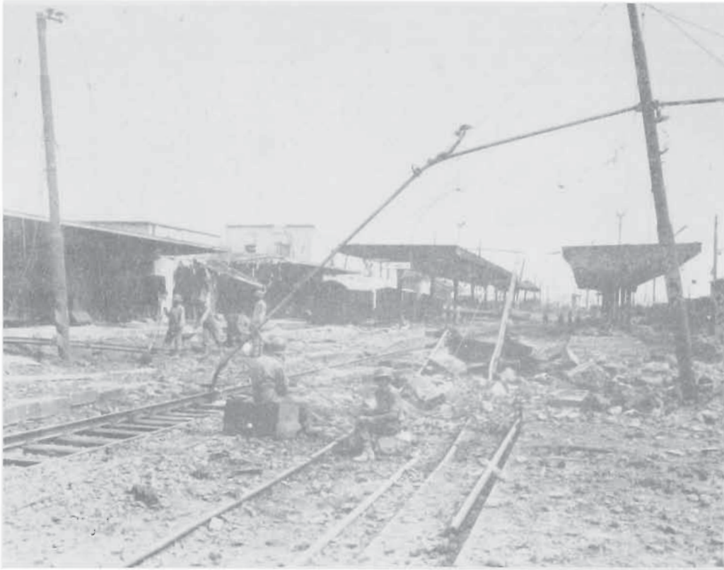
RAILROAD STATION AT BATTIPAGLIA
