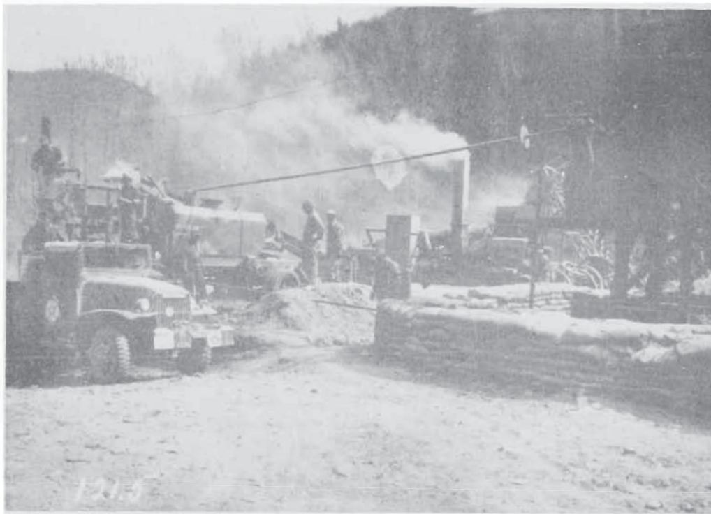
92ND ASPHALT MIX PLANT NEAR FUTA PASS
