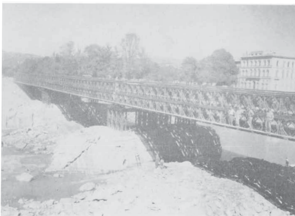
ARNO BRIDGE CONSTRUCTED BY 39TH
