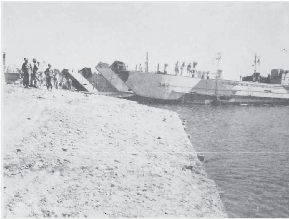
LCT HARDS BUILT BY 39TH AT PIOMBINO
