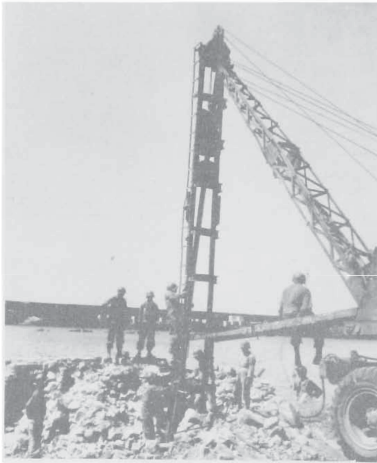
540th CONSTRUCTING PIER AT CIVITAVECCHIA
