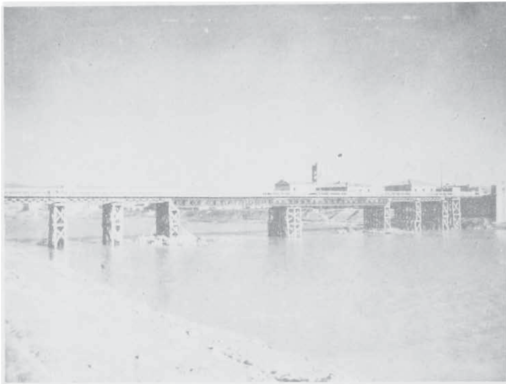
THE FINISHED BRIDGE
