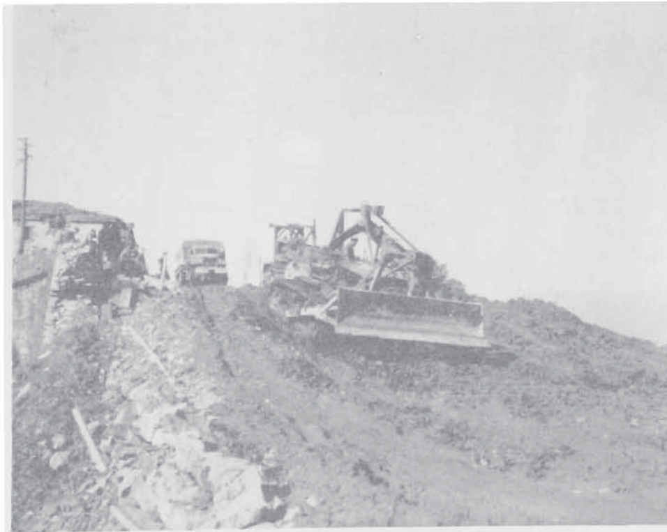
A 2750TH ANGLEDOZER WORKING NEAR VENTURINA
