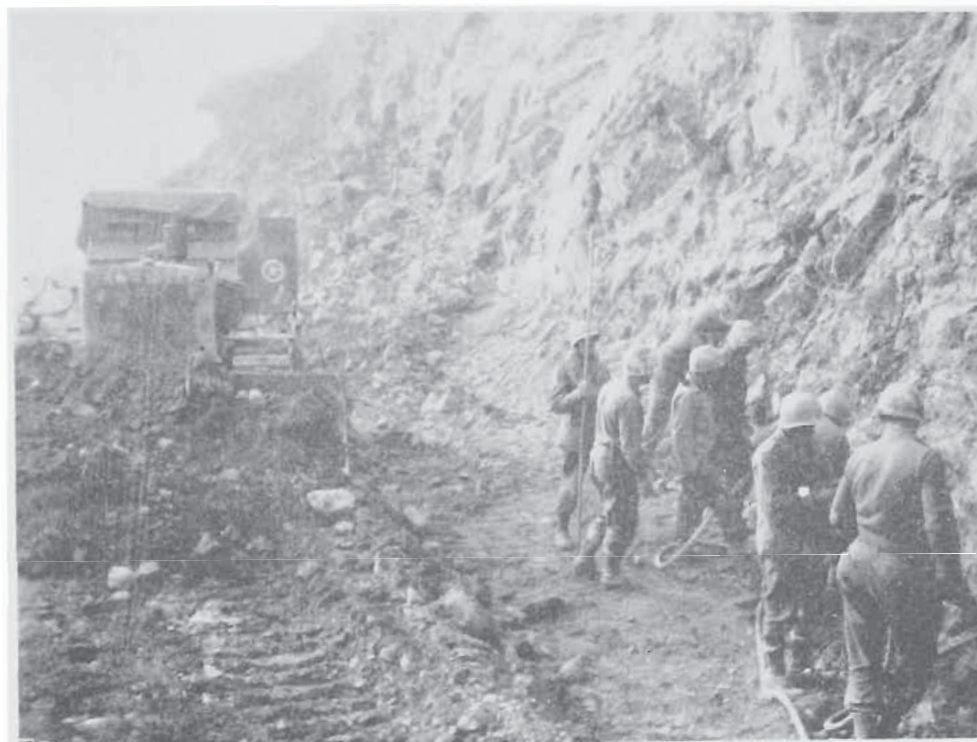
310TH PREPARING BLAST HOLES IN QUARRY NEAR BACCANELLO
