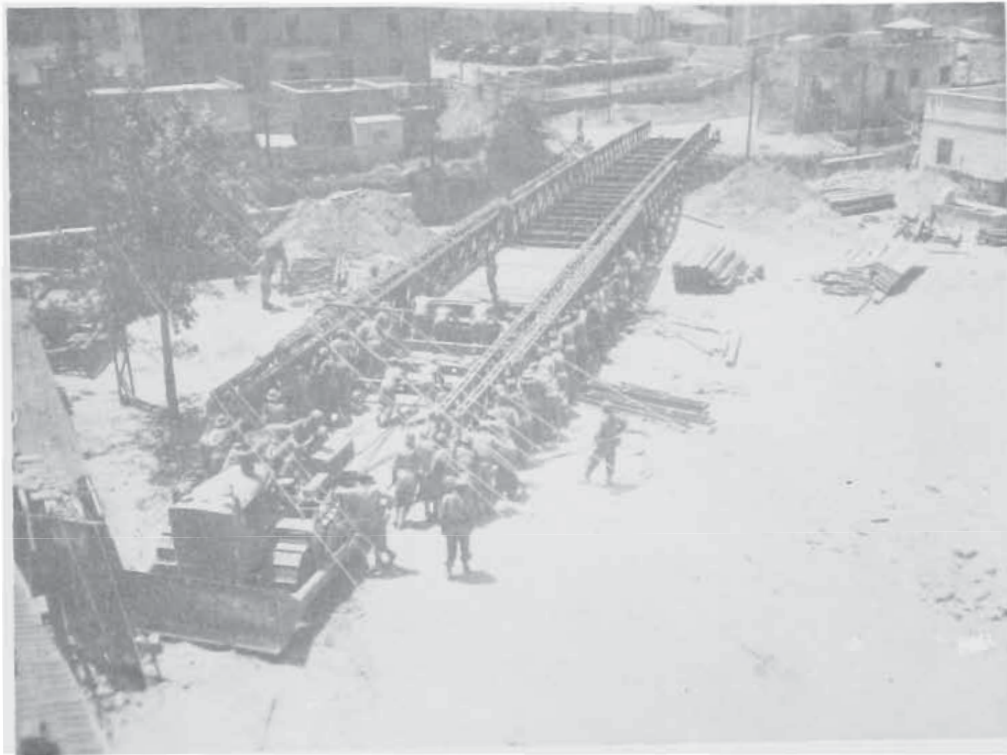
387TH LAUNCHING BAILEY AT CIVITAVECCHIA
