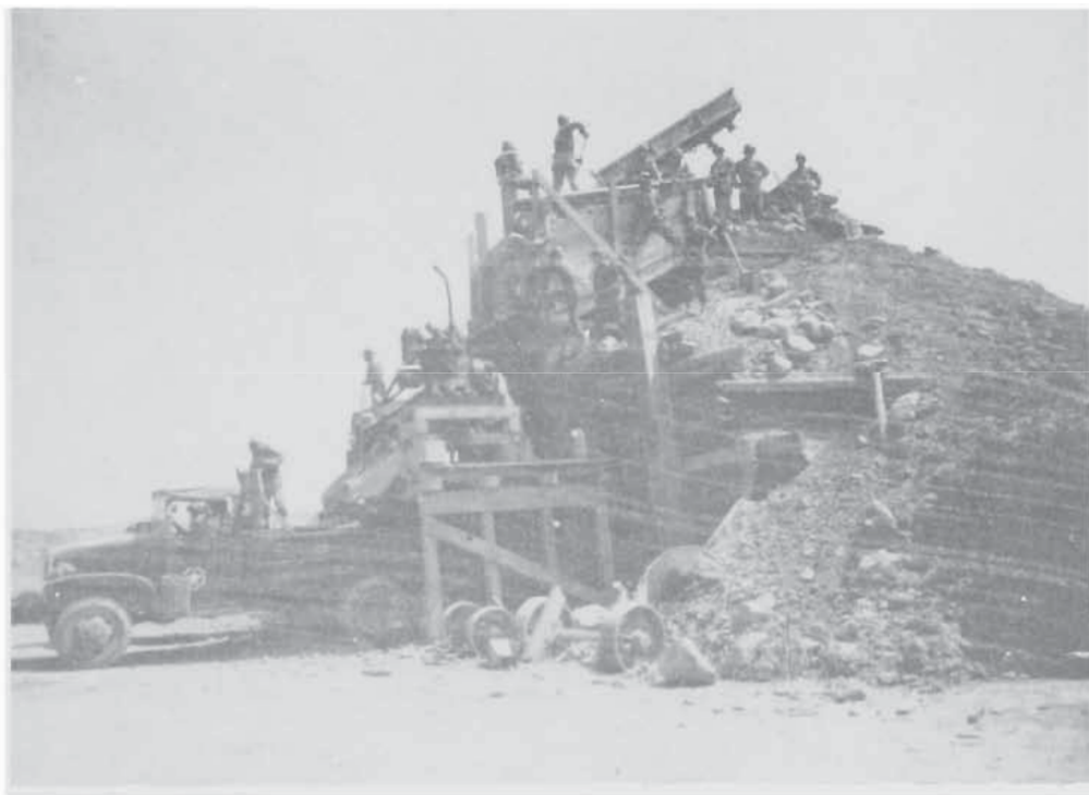
387TH OPERATING ROCK CRUSHER NEAR NETTUNO
