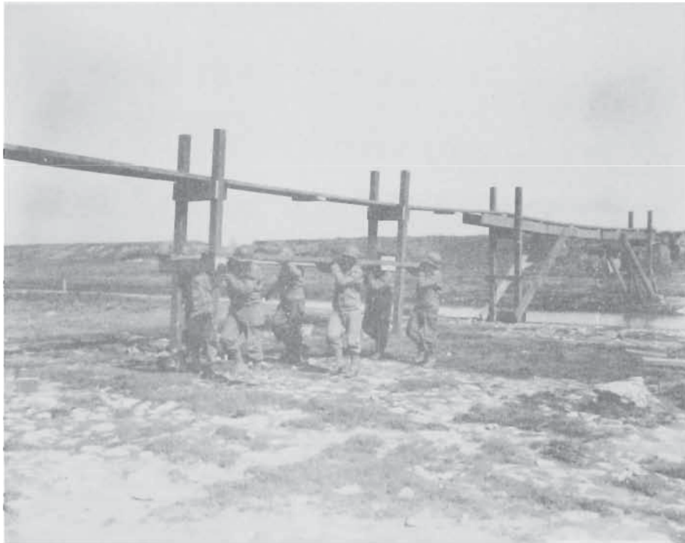
FOOTBRIDGE ACROSS MUSSOLINI CANAL BEING CONSTRUCTED BY 39TH ENGINEERS
