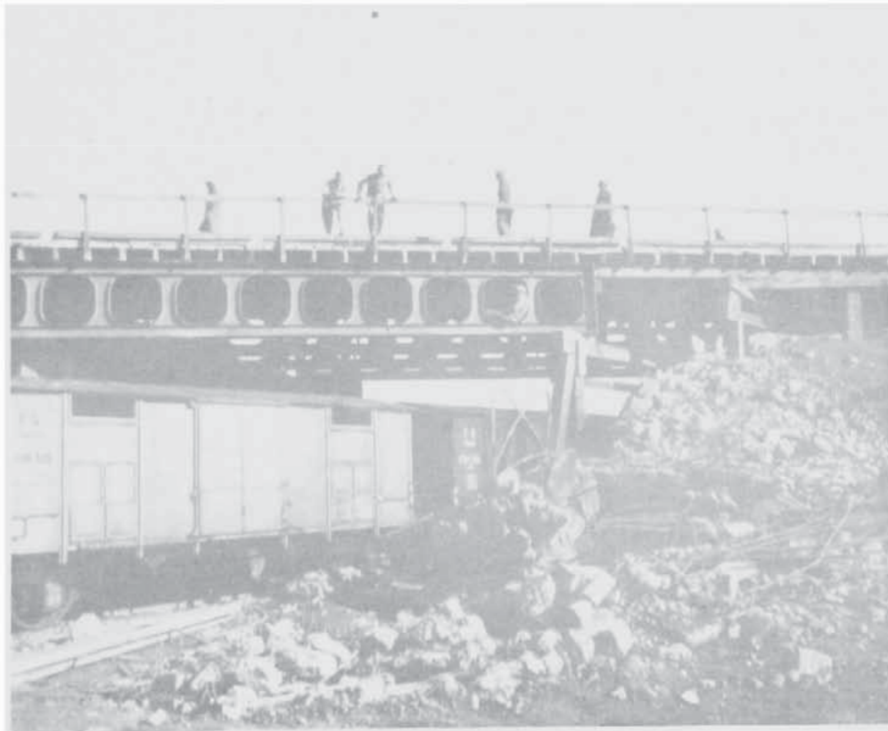
92ND ENGINEERS BUILDING OVERPASS NEAR CAPUA
