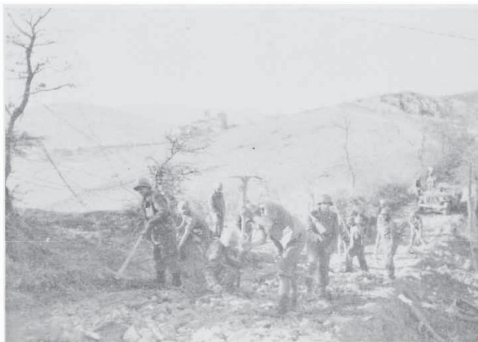
BRAZILIAN ENGINEERS BUILDING ROAD NEAR SILLA
