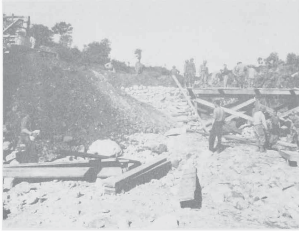
36TH ENGINEERS BUILD BRIDGE NEAR PRATA
