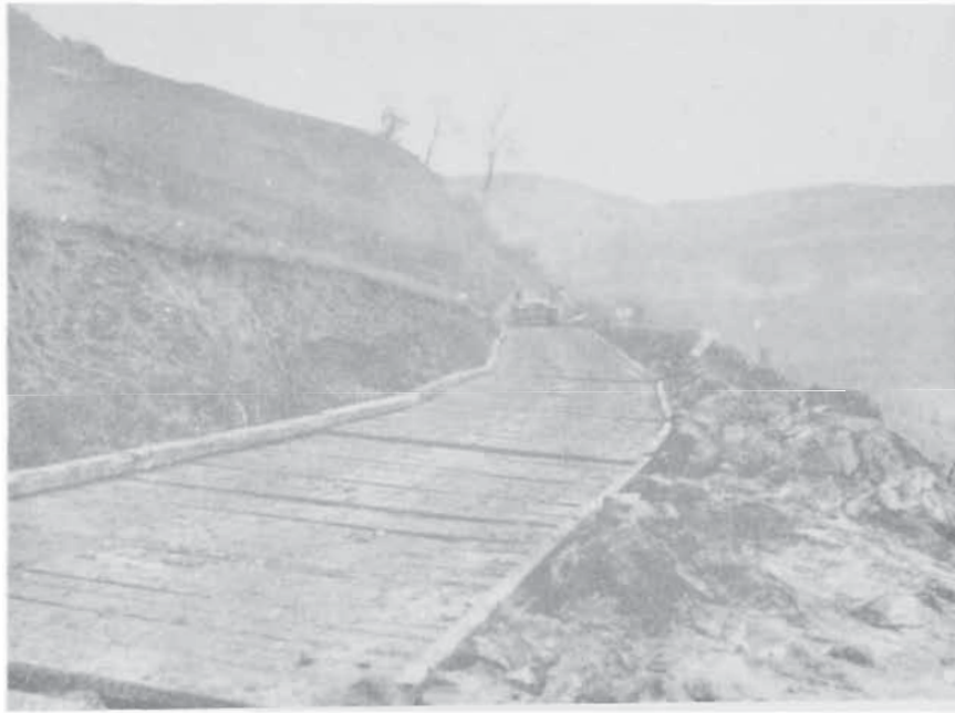
PLANK ROAD BUILT BY 109TH NEAR LOIANO
