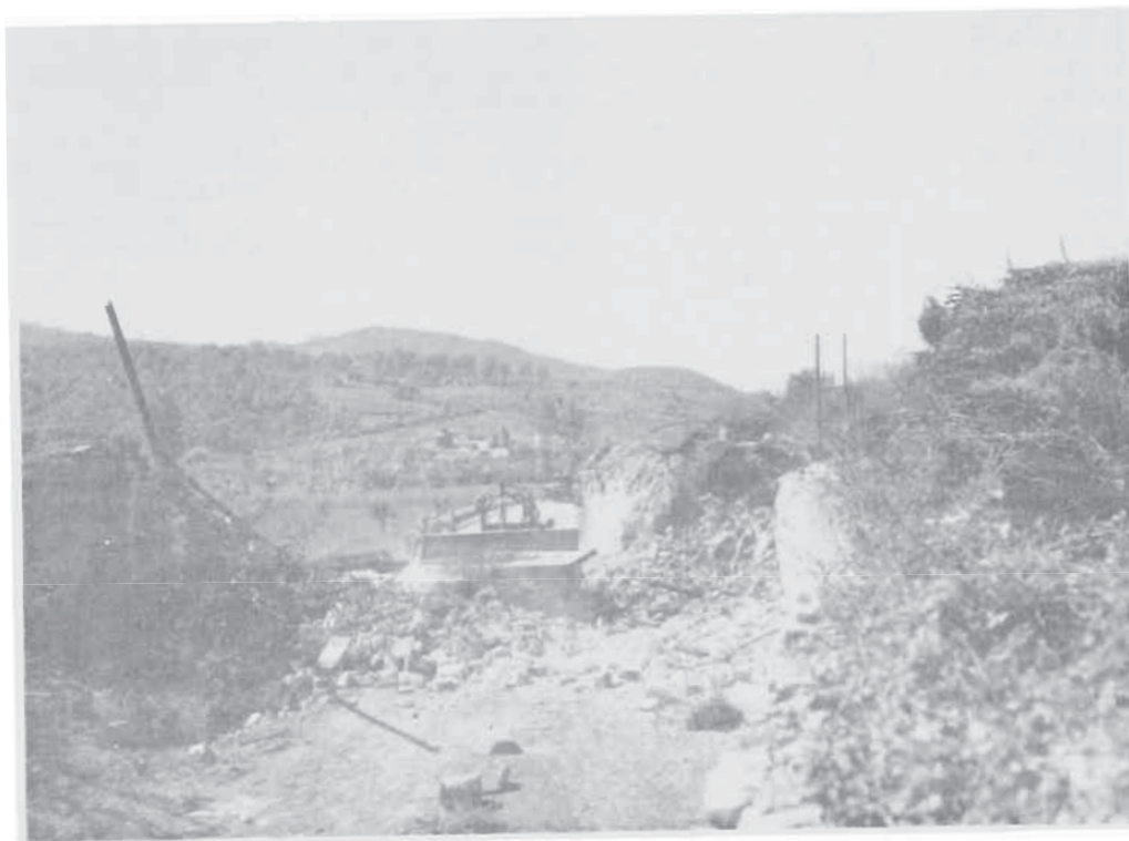
316TH CLEARING UP DEMOLISHED OVERPASS NEAR CAMPOMIGLIAIO
