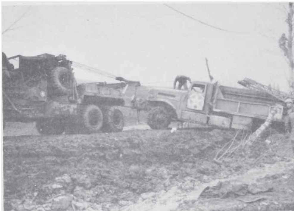
BRIDGE COMPANY BROCKWAY TRUCK IN DIFFICULTY NEAR S. BENEDETTO
