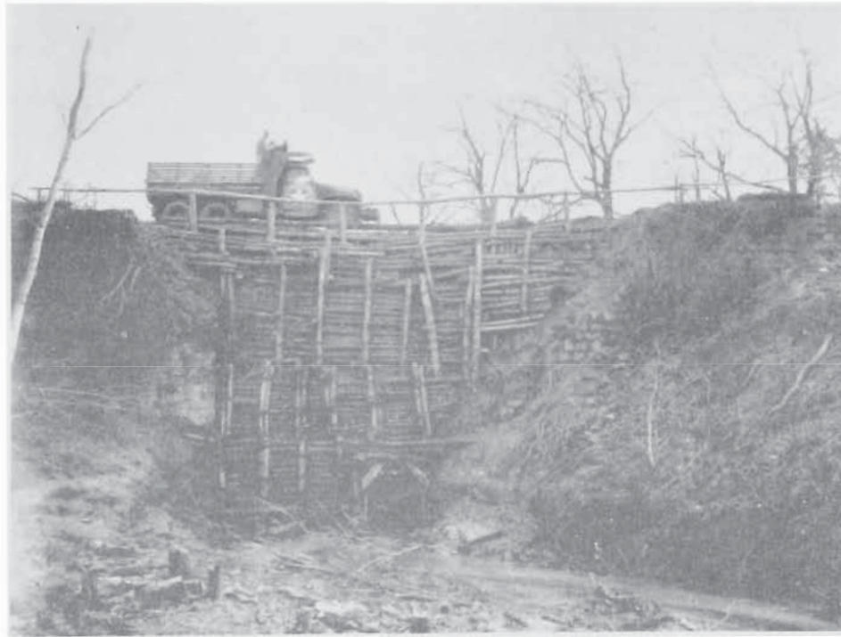
19TH ENGINEER CULVERT NEAR TEANO
