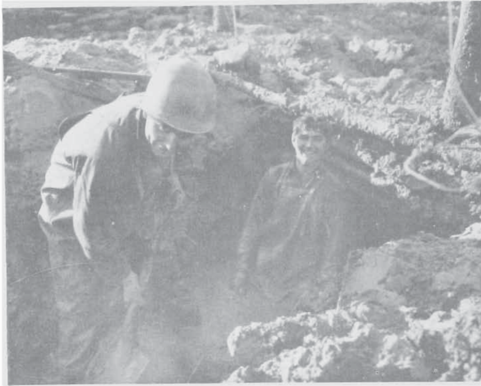
36TH ENGINEERS BUILDING CULVERT AT MONTAQUILA
