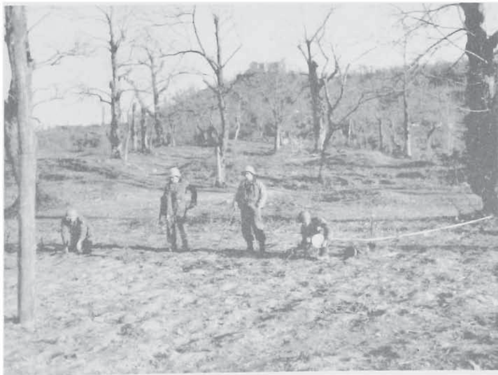
BRAZILIAN ENGINEERS MARKING A GERMAN MINEFIELD NEAR MOUNT CASTELLO
