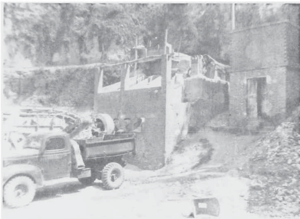
TRUCK OF BRITISH 3RD AIRFIELD CONSTRUCTION WAITING FOR A LOAD OF GRAVEL NEAR PIETRASANTA
