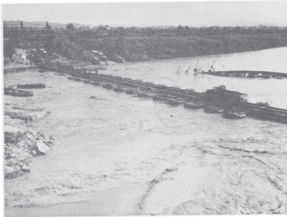
BRIDGE AT PONTEDERA CONSTRUCTED BY 16TH ENGINEERS
